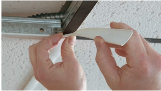
Applying GridMax Over T-bar Suspension Grid System
