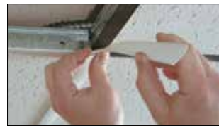
Applying Gridmax over T-bar suspension grid system
